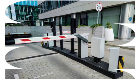
Entrance gates and factory access roads
